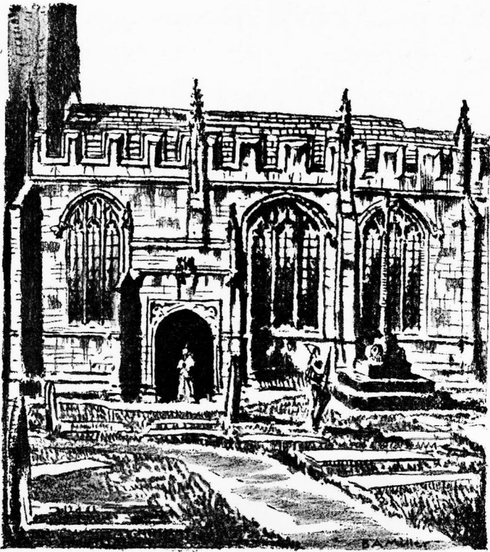
Gawsworth Church. The South Porch.
